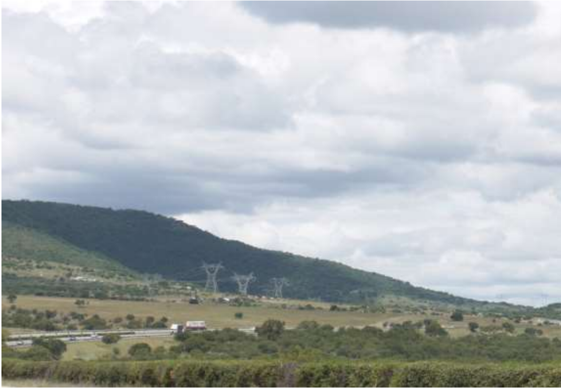
Plate 13 - Existing 400kV double overhead transmission lines. Pylons are obvious in the mid distance (approximately 2-3km) but are not highly conspicuous at a distance (approximately 5-6km) as they cross the ridgeline.
