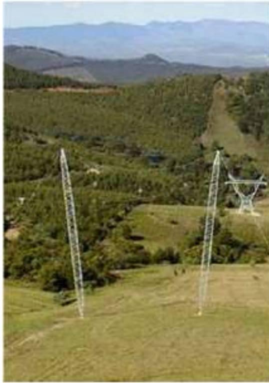
Figure A-2: Tower Type 524 (Cross Rope).
